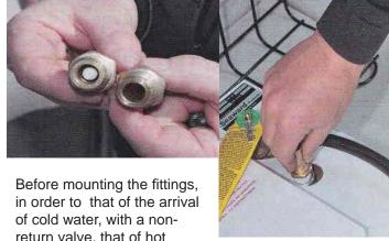
in order to that of the arrival of cold water, with a non-return valve, that of hot water outlet that does not have, and seal the connector threads with the help of Teflon tape.
